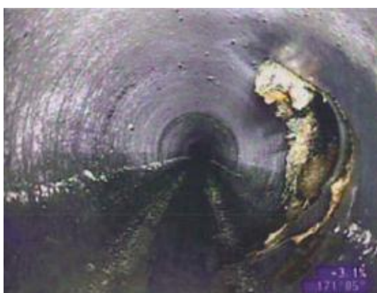
Mineral Deposits at Service Connection (no boot/wye)
