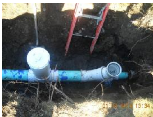
PVC Cleanout (similar to wye, minimizes leaks)
