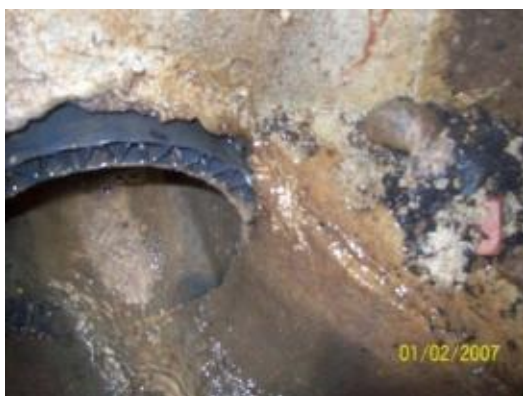
MH 3-15 pipe-MH joint leak (no boot/seal)
